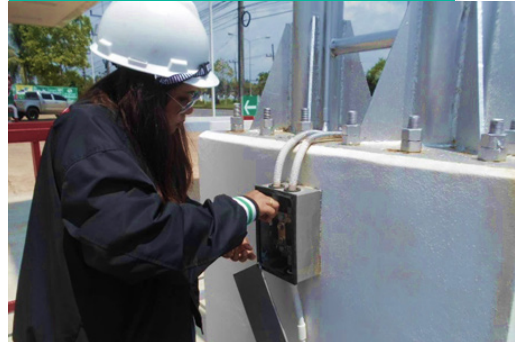
Inspections and Gas Station Safety and Environment Training
